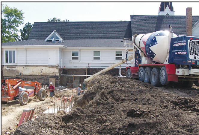
Concrete is poured for the the new footings.
